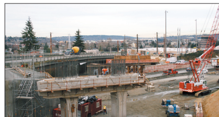
I-405 | Work on improvements to Interstate 405 near Renton City Hall are six to nine months ahead of schedule [3]
