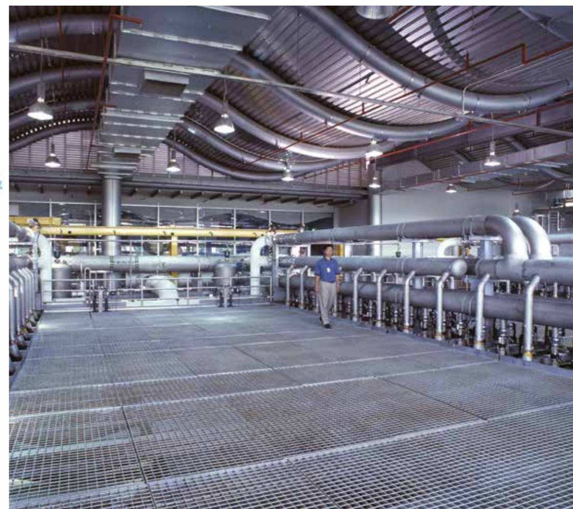
Left: The city of Abilene, Texas, uses Suez’s ZeeWeed ultrafiltration hollow-fiber membranes technology to treat any raw water to the quality needed
