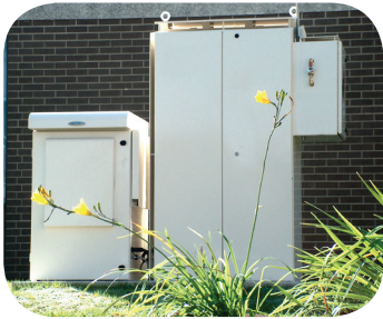
This GenCore is used to generate electricity to power the telephone system at our Latham facility in the event of a grid power failure.
