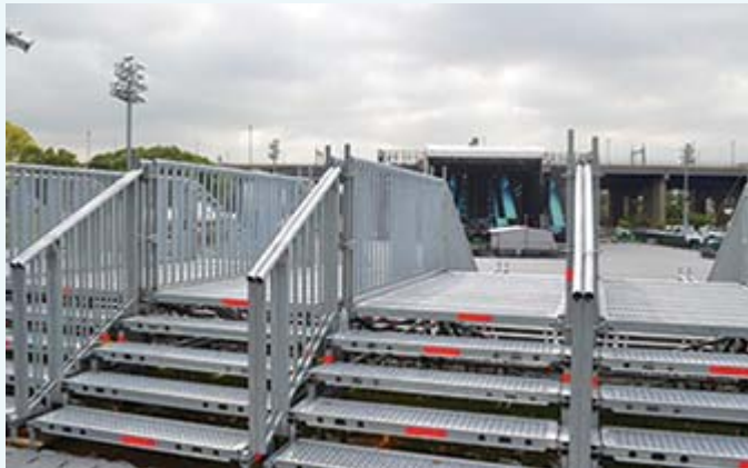
Reduced stair heights, wider tread, lock-in decks, and guardrails are among the safety features designed to minimize the possibility of slips, trips, and falls in heavy foot traffic.
