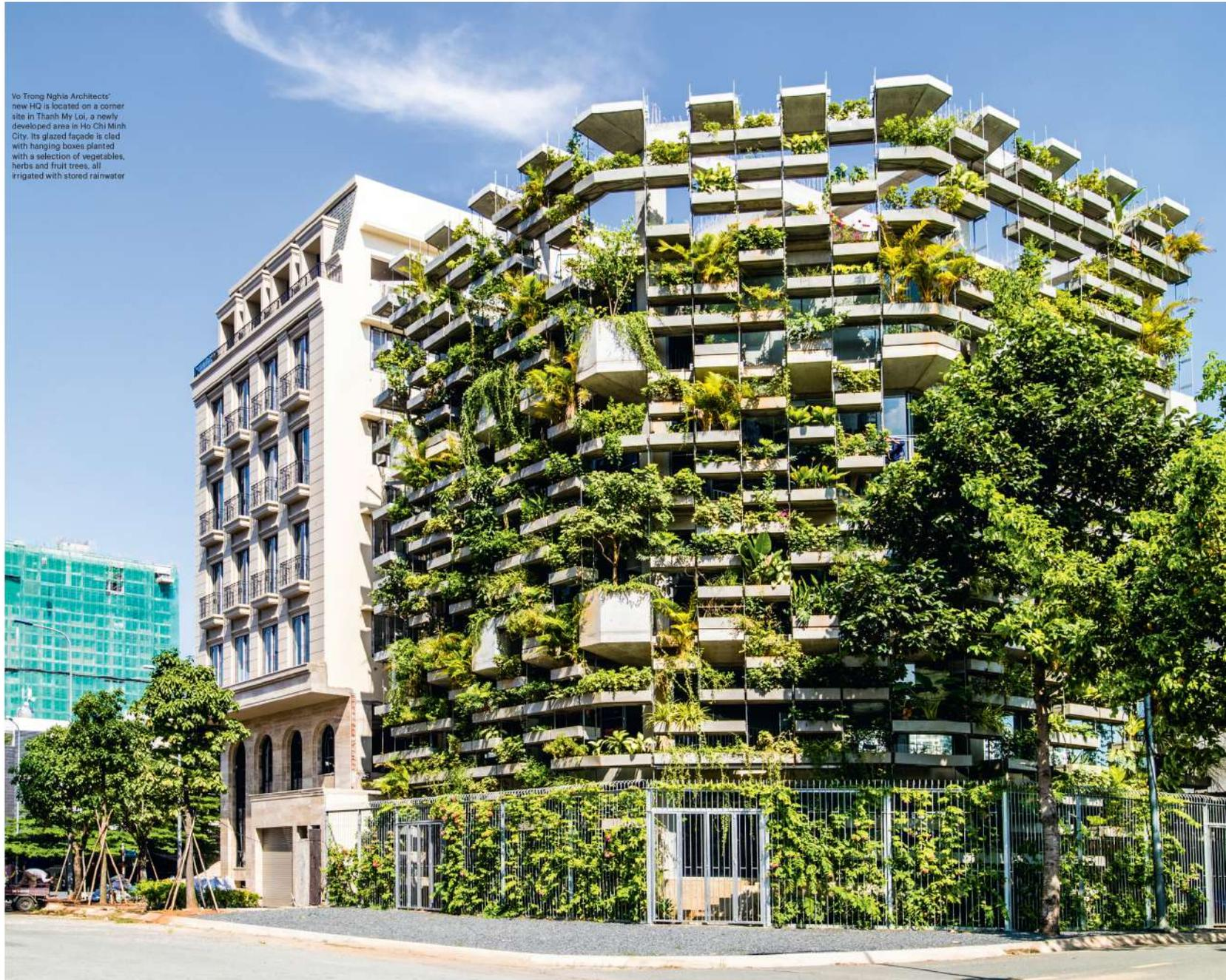
Right, the ground floor of the architects' HQ. The building's planted green curtain filters direct sunlight and purifies air, while the water evaporating from its irrigation system helps keep the rooms cool
