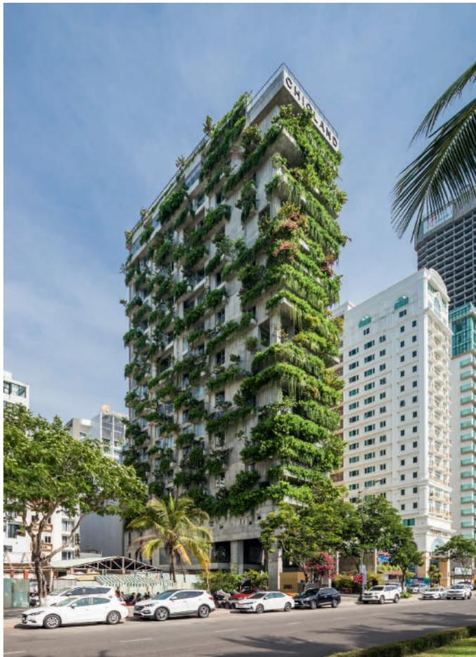
allow the buildings to look after themselves.' In the rainy season, which in Ho Chi Minh City lasts for half the year, tropical downpours water the plants every day. The office also collects water and channels it to the basement, where it is stored and pumped to the concrete plant troughs during the dry season. A gardener needs to inspect and treat the plants for diseases only a handful of times a year.
