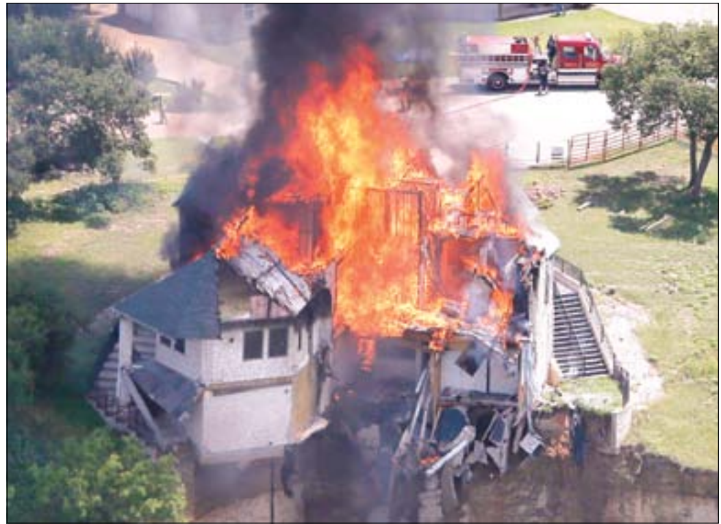
Smoke rises from a house deliberately set on fire, days after part of the ground it was resting on collapsed into Lake Whitney, Texas. Building crews set fire on Friday to the luxury lake house left dangling about 75 feet on a decaying cliff that has been giving way underneath the structure.
