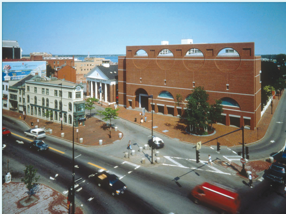
Charles Shipman Payson Building, Portland Museum of Art, view from Congress Square. Photo: Craig Becker.
