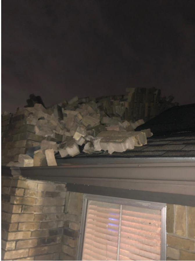
The chimney of Shelby's house collapsed as the tornado ripped through the street.
