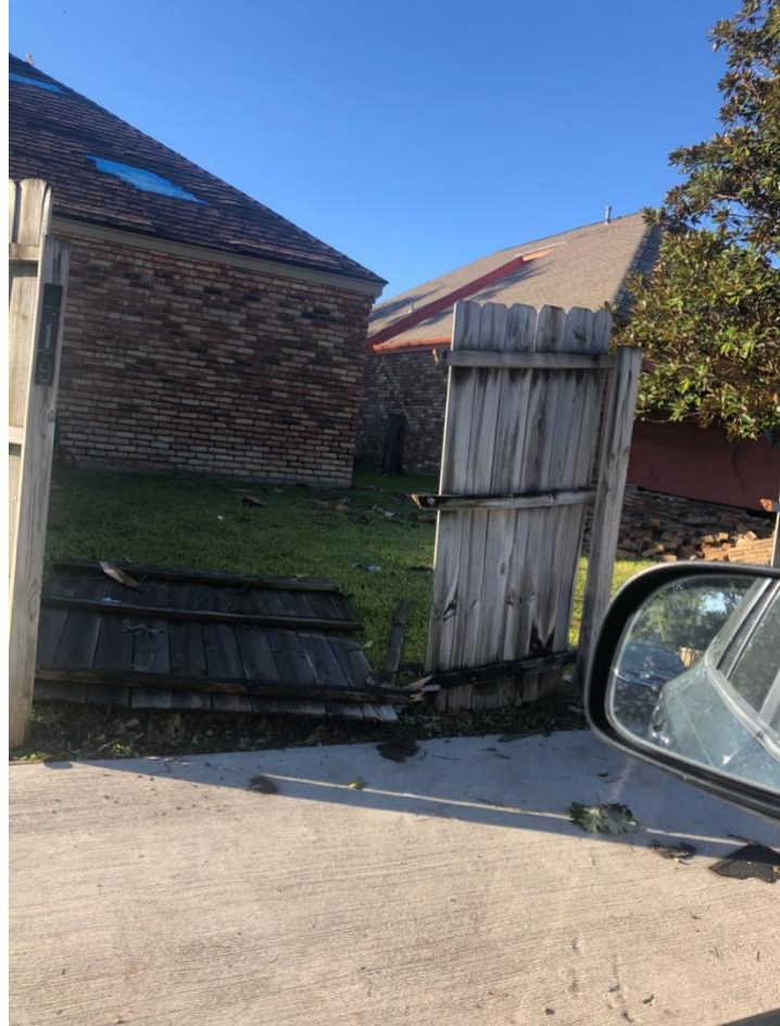
Fences were destroyed after the Oct. 20 tornadoes.
